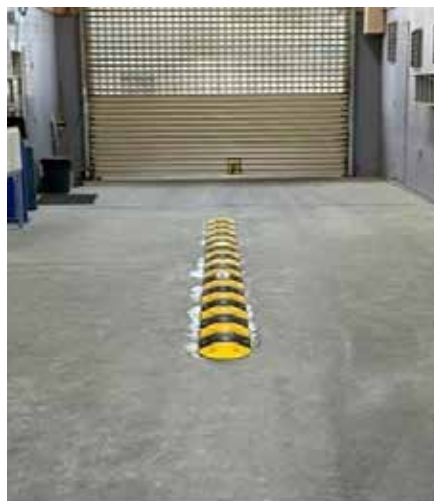
Sensors housed in speed bumps permanently affixed to the search area surface
